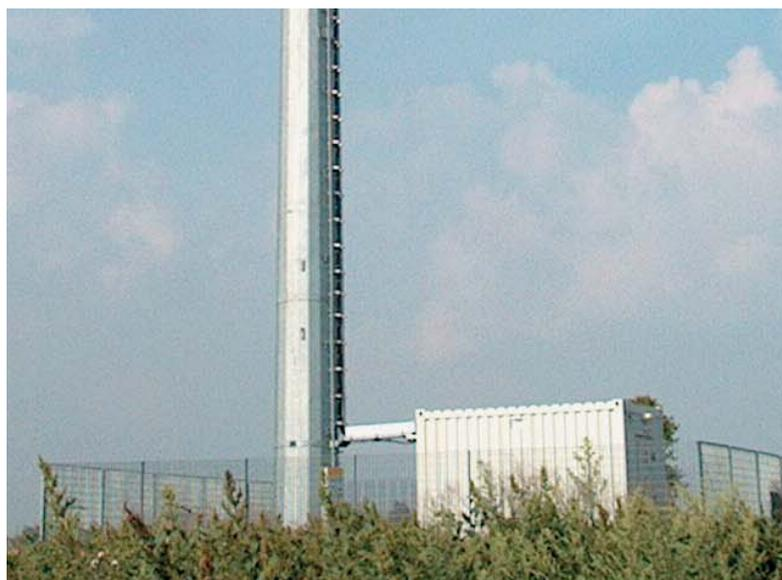
The particularly slender shape, the assembling simplicity and quickness as well as the cheaper prices compared with the lattice works, made it possible that the monotubular steel column found a wide application in the field of telecommunications. The experience gained in designing and manufacturing such supports, proposes ourselves as qualified suppliers among the bigger Italian companies in this field.
